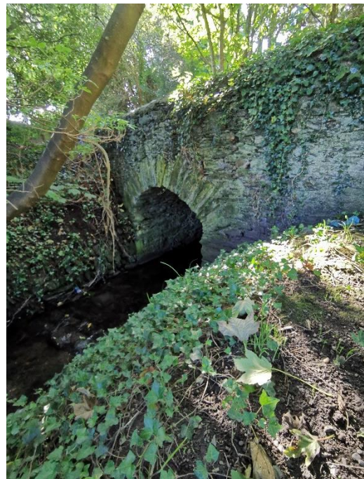
Photograph 32: Stone arch bridge
