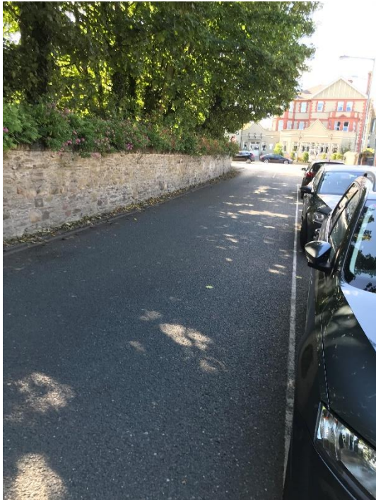
Photograph 37: Boundary wall looking up Wentworth Place towards Abbey Street
