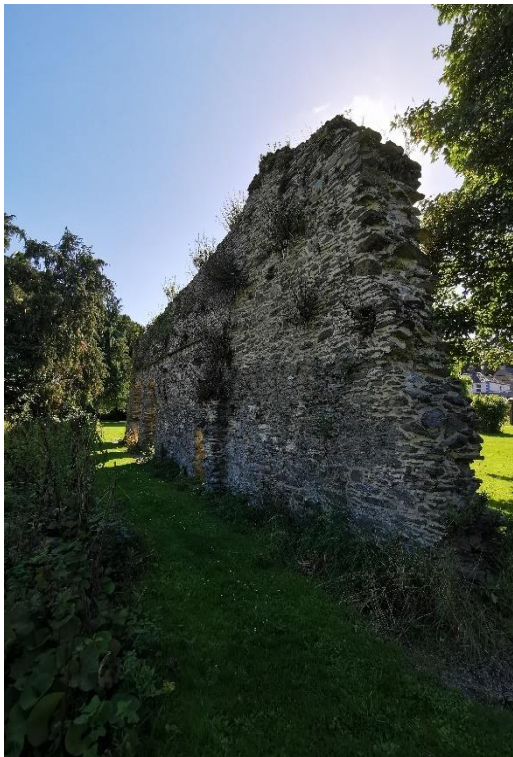
Photograph 7: Northern Friary wall with vegetation growth
