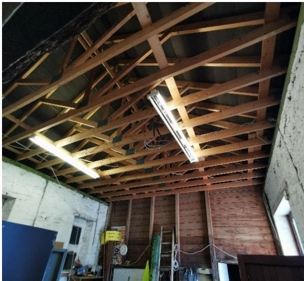
Photograph 15: Modern truss rafter roof
