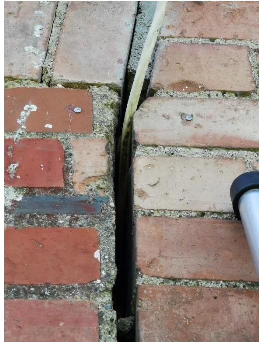
Photograph 26: Crack monitoring pip location 5
