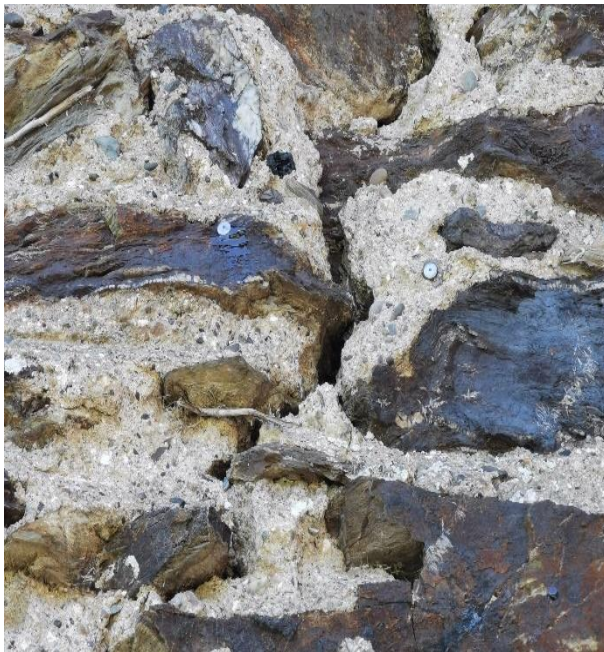
Photograph 21: Crack monitoring pips location 1
