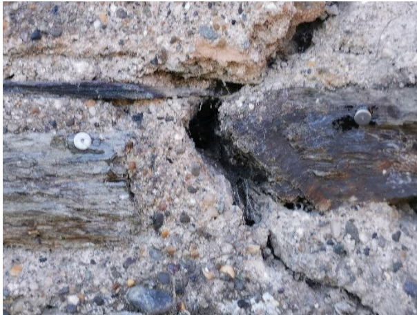
Photograph 21: Crack monitoring pips location 1
