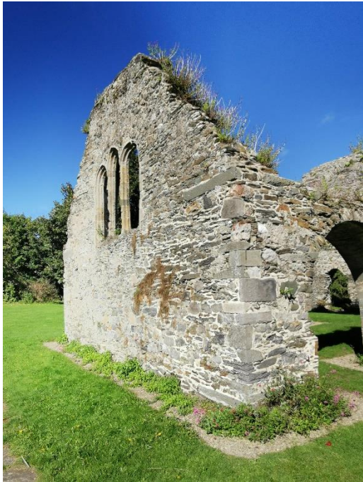
Photograph 1: Southern Gable wall to Friary
