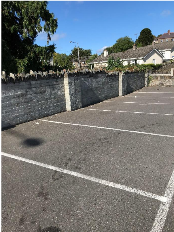
Photograph 35: Blockwork boundary wall with stone capping within car park
