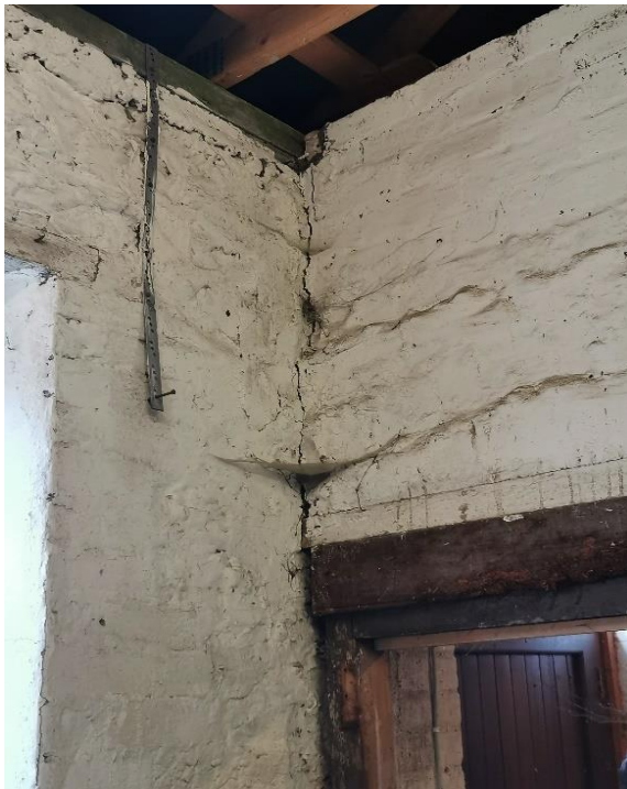
Photograph 11: Separating of internal wall from external wall
