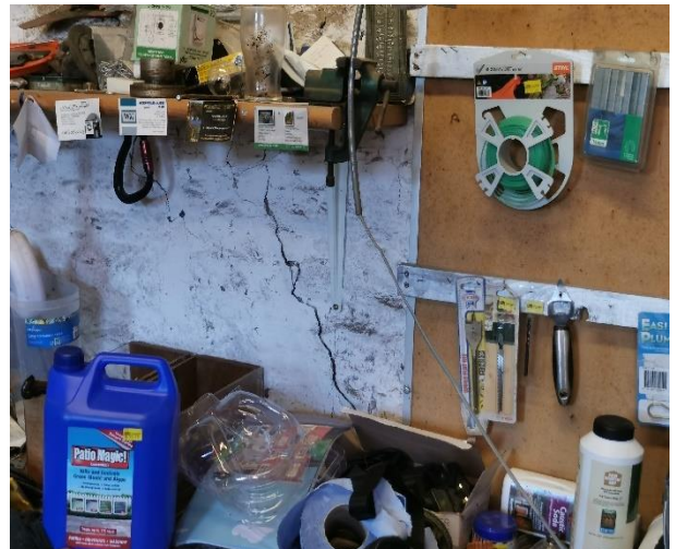
Photograph 10: Crack at weakest point in wall
