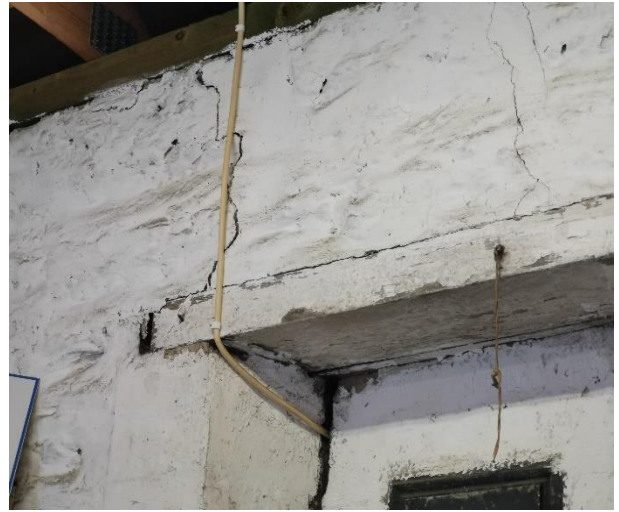
Photograph 10: Crack at weakest point in wall
