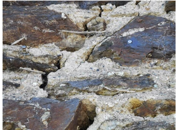
Photograph 22: Crack monitoring pips location 2
