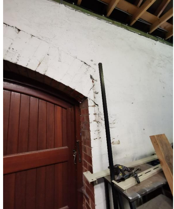
Photograph 18: Masonry dislodged
